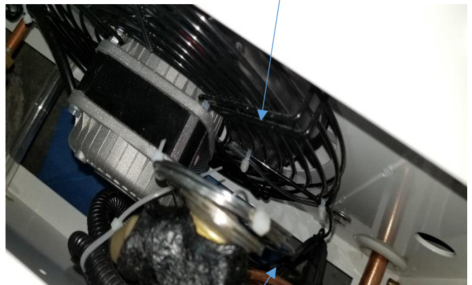
Defrost Suction Line Sensor (PB2)
