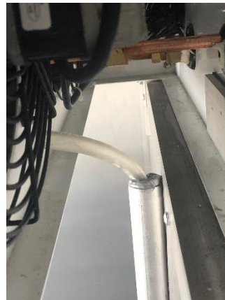
Drain Tube in evaporator
